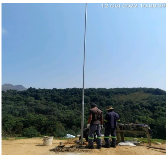
Installation of lightning conductors in October 2022
