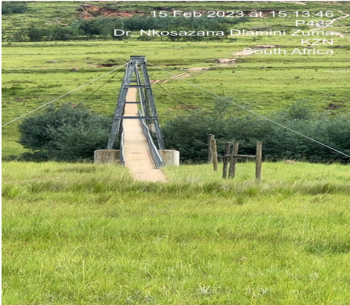
Pedestrian Bridge in Dr. Nkosazana Dlamini Zuma Municipality
