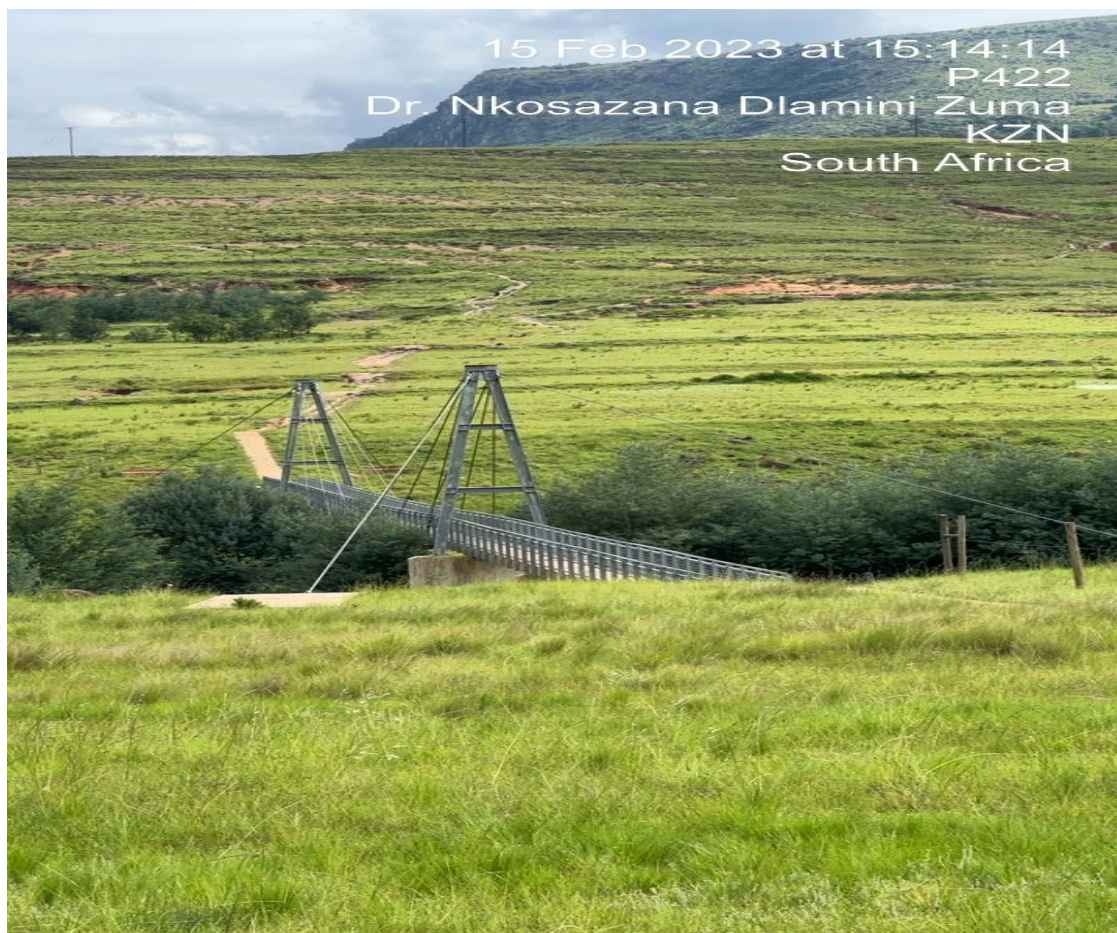
Pedestrian Bridge in Dr. Nkosazana Dlamini Zuma Municipality
