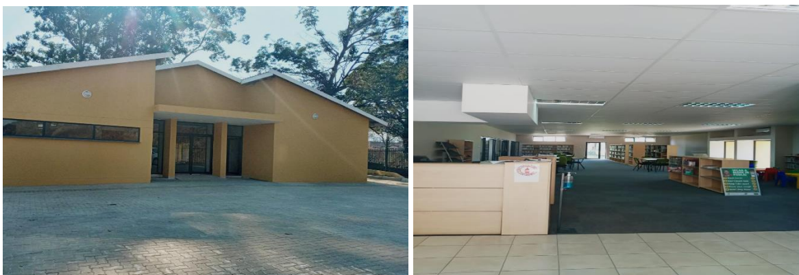
Figure 14, New Creighton Library
