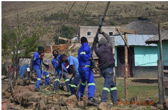
Installation of lightning conductors
