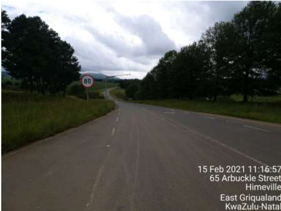
Camera at Sani Pass Intersection
