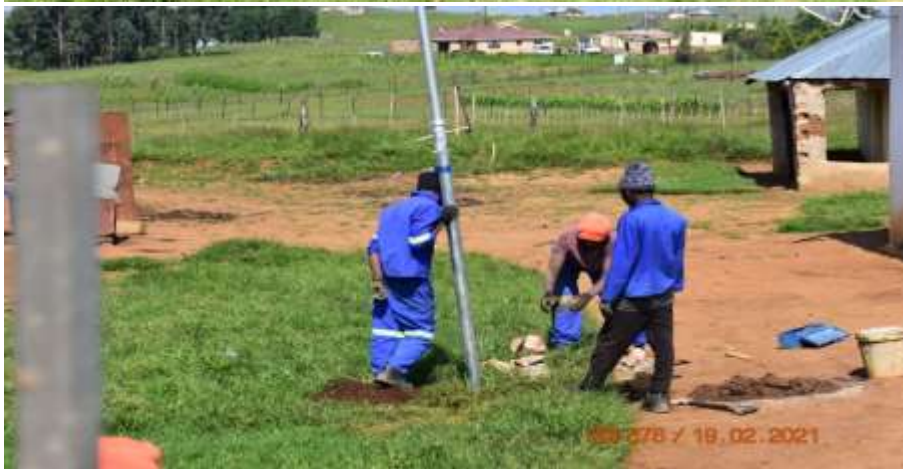
Installation of lightning conductor
