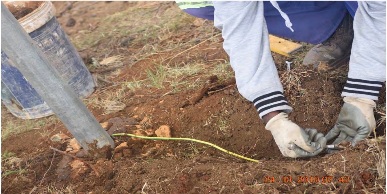
Installation of lightning conductor
