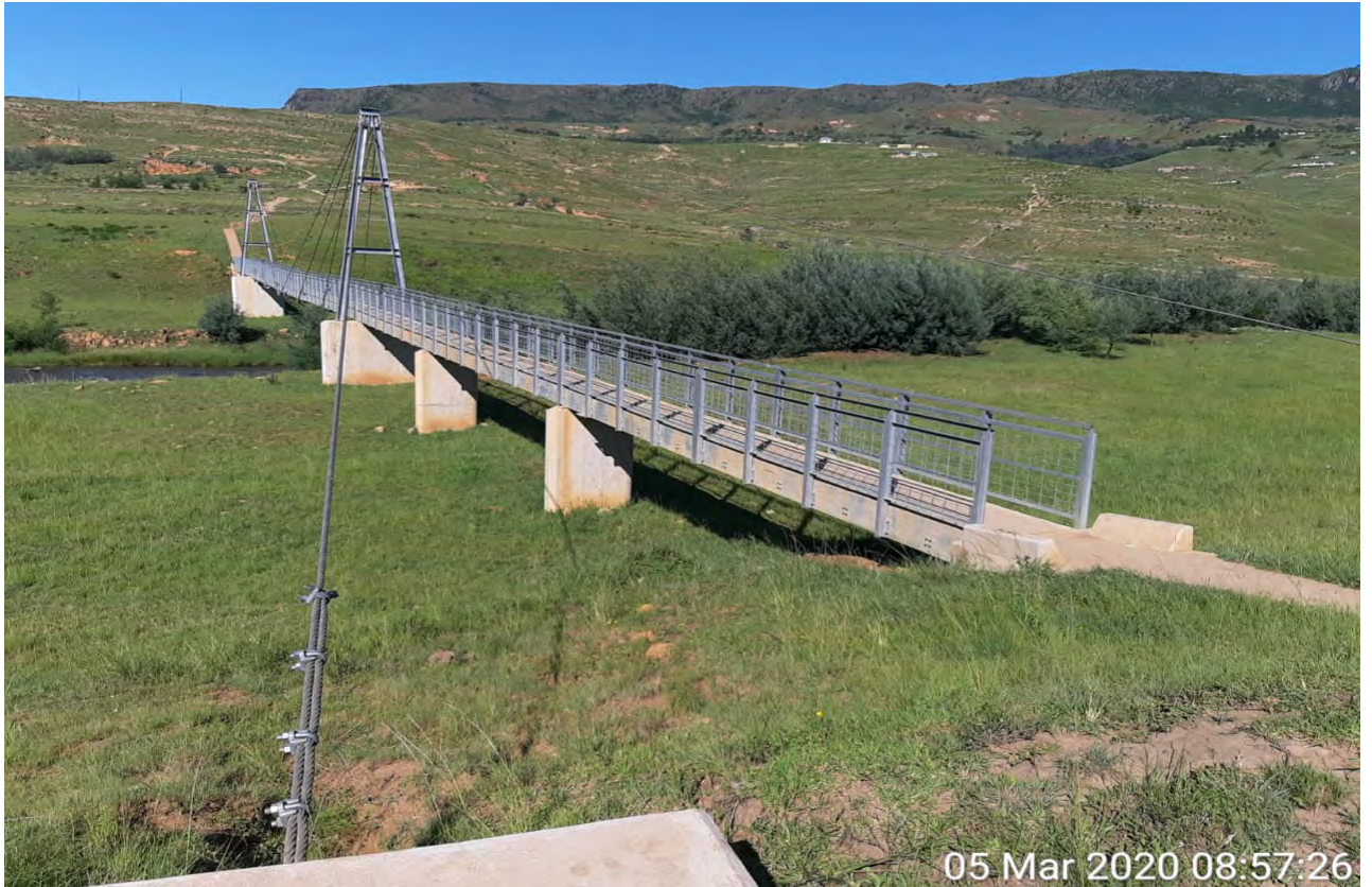
Pedestrian Bridge in Dr. Nkosazana Dlamini Zuma Municipality
