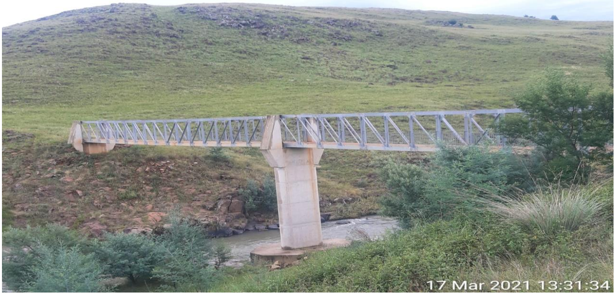
Ward 1 Pedestrian Bridge Emhlangeni- KwaZinkwana
