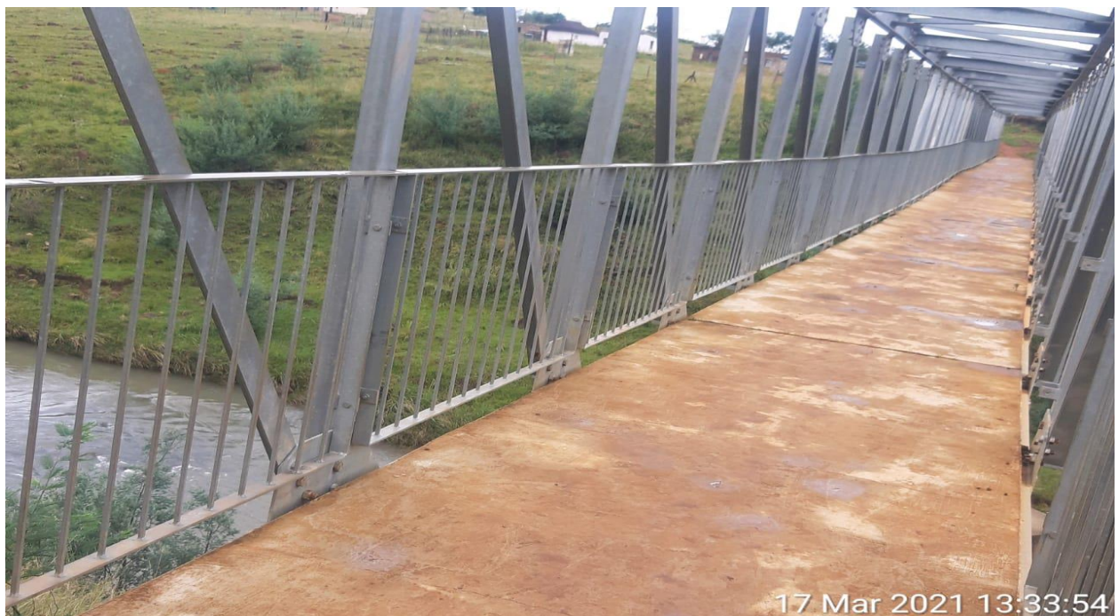
Pedestrian bridge ward 1 Emhlangeni EMHLANGENI KwaZinkwana
