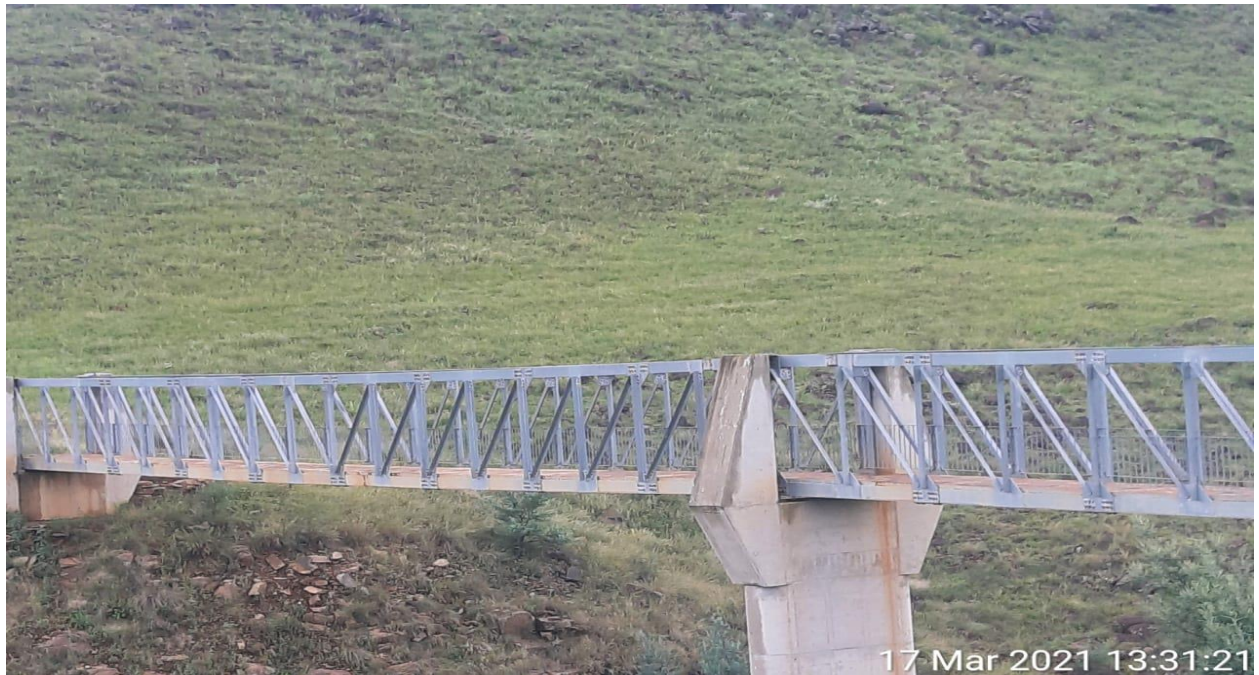
Pedestrian Bridge in Dr. Nkosazana Dlamini Zuma Municipality
