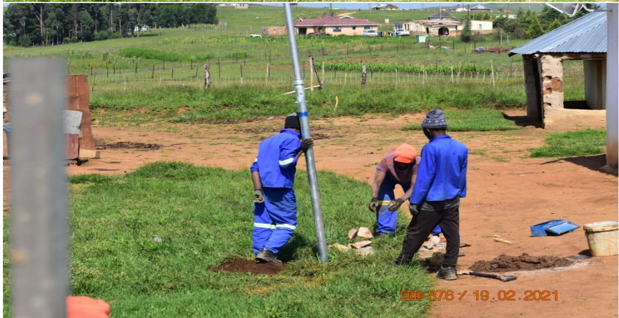
Installation of lightning conductor
