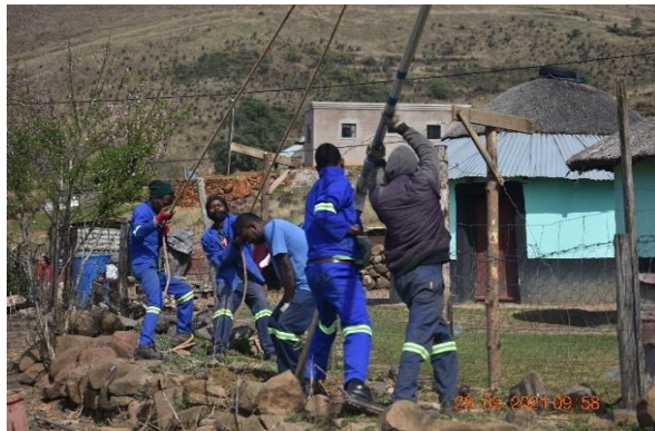
Installation of lightning conductors
