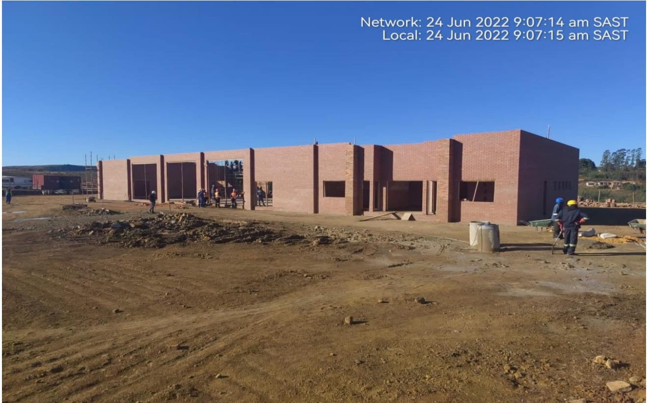
Current picture of the Dr. NDZ Emergency Centre in Bulwer
