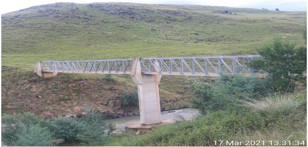
Ward 1 Pedestrian Bridge Emhlangeni- KwaZinkwana
