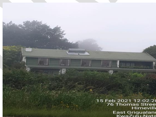
One of the houses in the Himeville Suburbs that utilizes Solar energy
