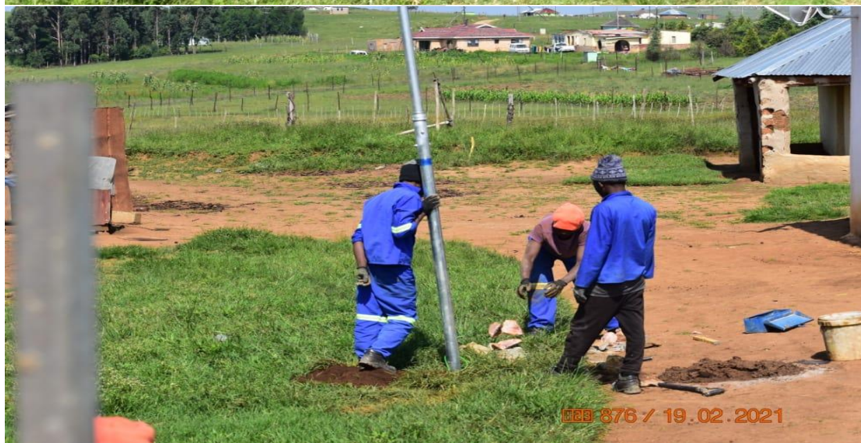
Installation of lightning conductor
