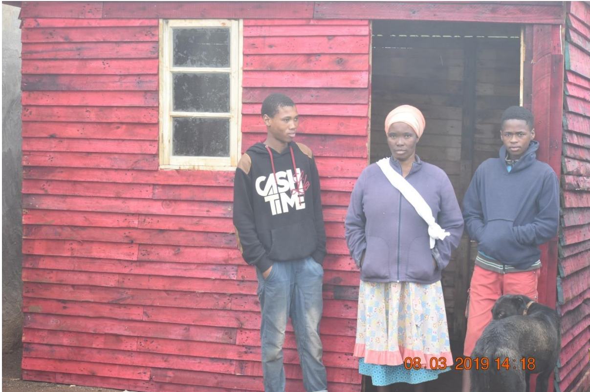
Figure 31- An emergency house provided to a family affected during the February- march 2019 heavy rains
