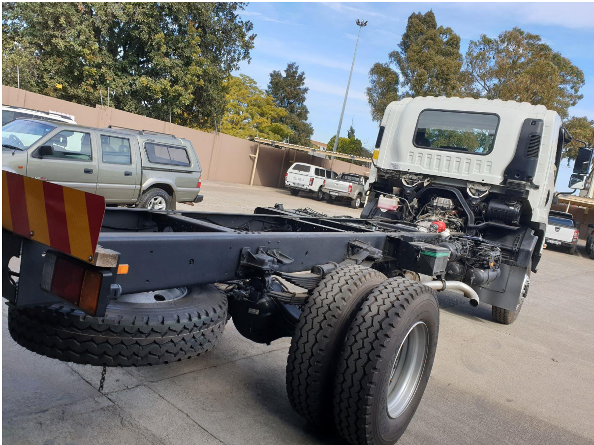
Figure 9 – Rear part of the cab where the superstructure of the fire truck will be installed
