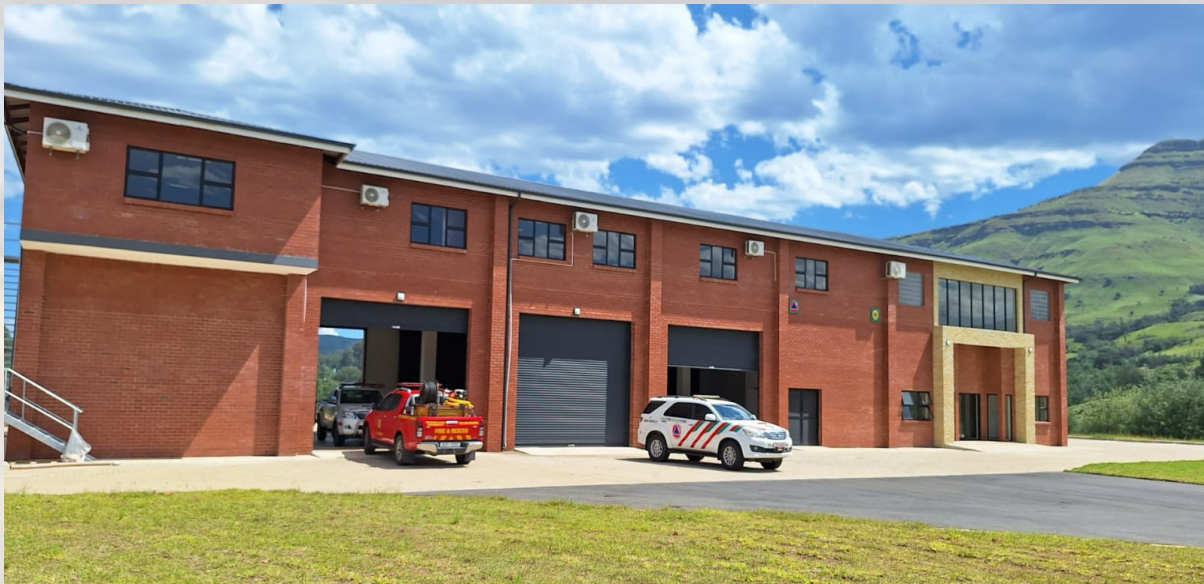
DR. NDZ Disaster Management Center located in Bulwer along the R617
