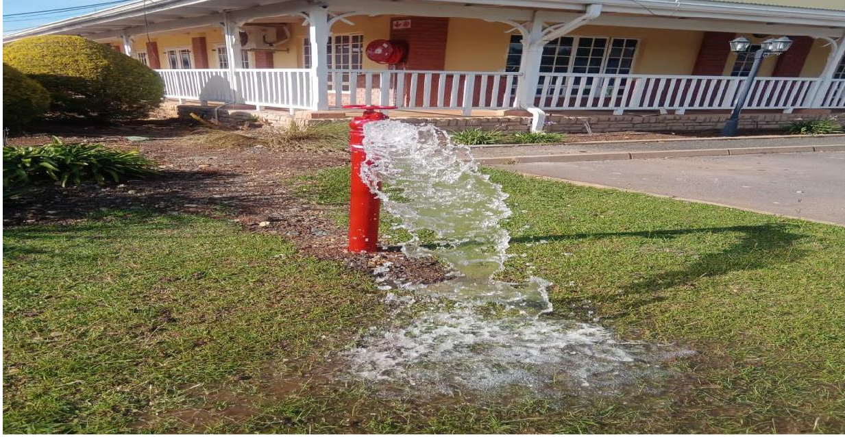
Pressure Testing Stage of Fire Hydrants.
