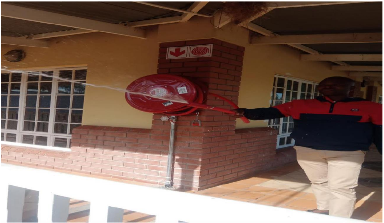
Pressure testing of Fire hose reel.
