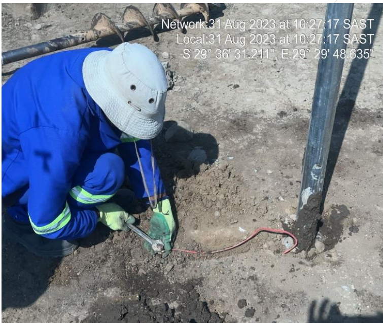
Installation of Lightning Conductors in August/ September 2023
