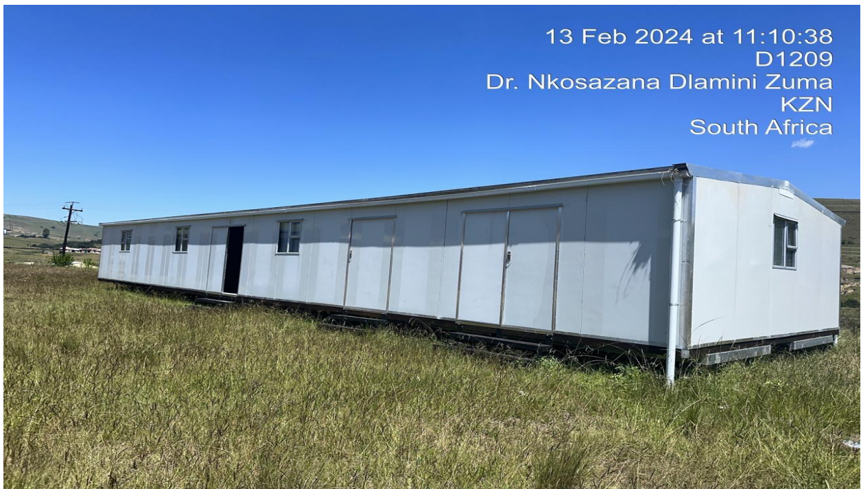
Park home for fire satellite station constructed in ward 12
