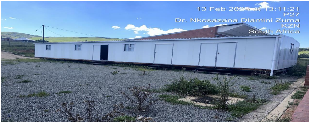
Park home for fire satellite stations constructed in ward 1
