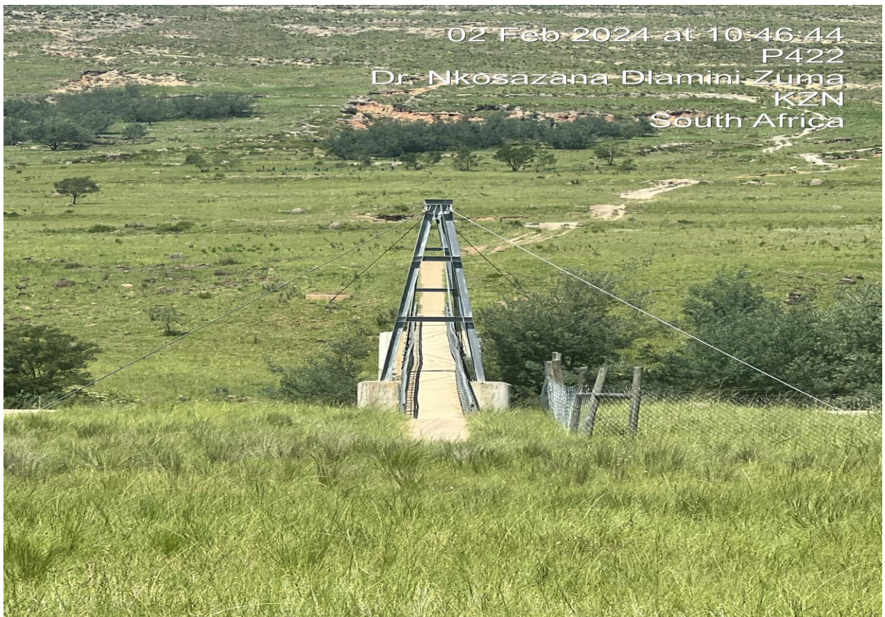
Pedestrian Bridge in Dr. Nkosazana Dlamini Zuma Municipality
