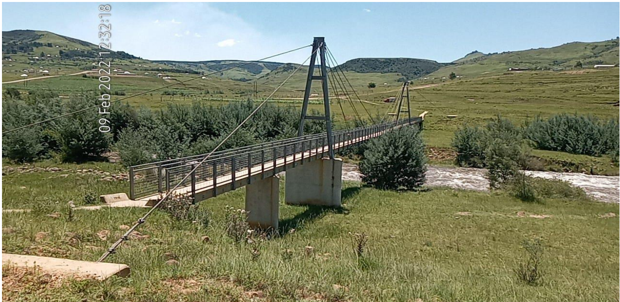
Pedestrian Bridge in Dr. Nkosazana Dlamini Zuma Municipality
