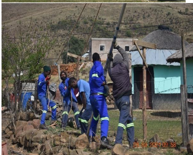
Installation of lightning conductor
