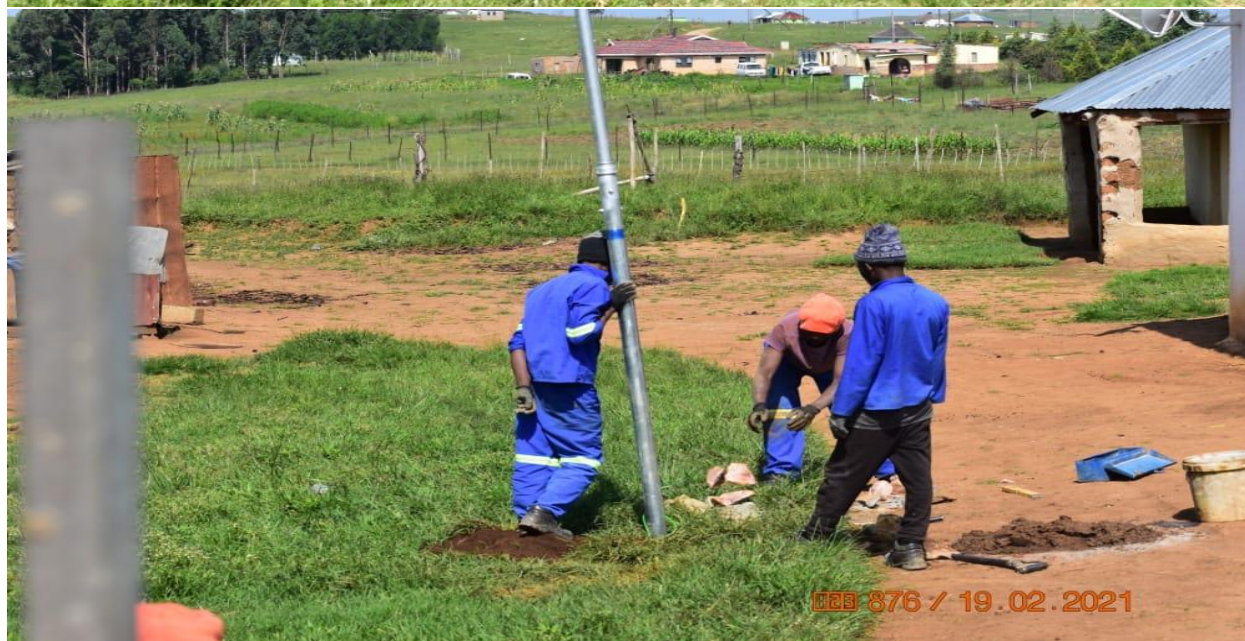
Installation of lightning conductor
