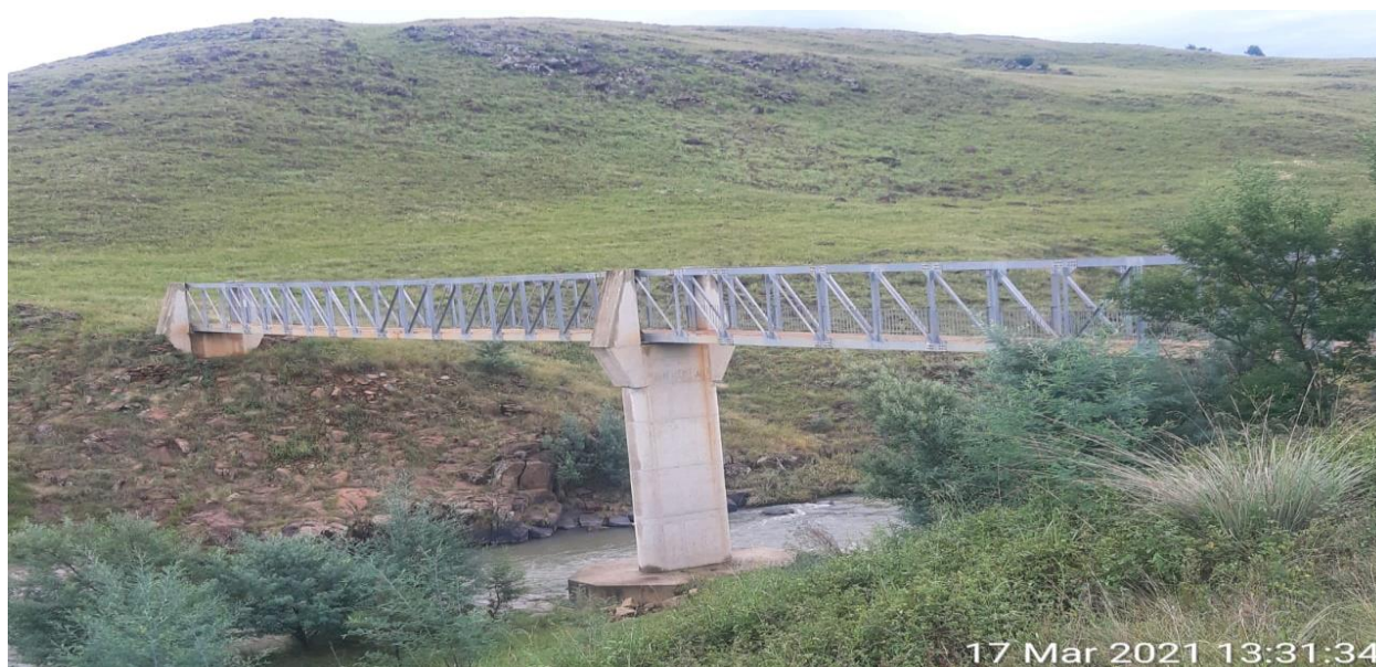
Ward 1 Pedestrian Bridge Emhlangeni- KwaZinkwana
