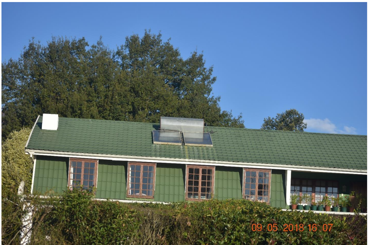
One of the houses in the Himeville Suburbs that utilizes Solar energy
