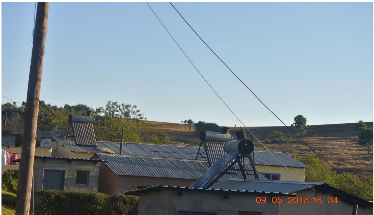
Solar gysers at Himeville Township
