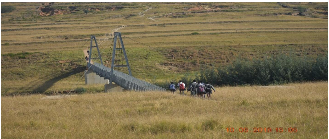
Pedestrian Bridge in Dr. Nkosazana Dlamini Zuma Municipality
