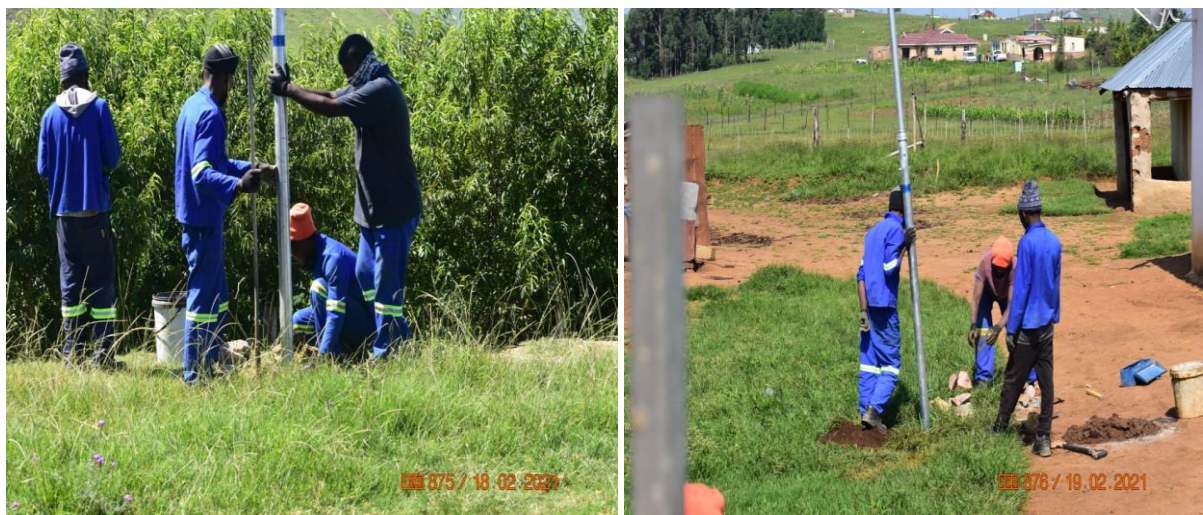
Figure 11- Lightning Conductors being Installed
